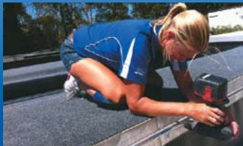
2. Fitting Lower Aluminum Sailtrack
