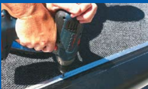
4. Fitting top Sailtrack onto Fender
