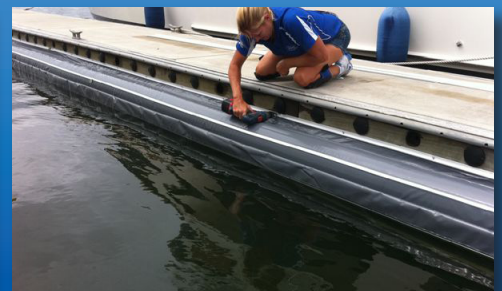
4. Fitting Super Fender lower track 90mm from top
