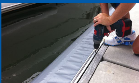
5. Fixing Top Flap of Super Fender onto Pontoon
