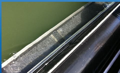
3. Super Fender laying alongside pontoon ready for fitting
